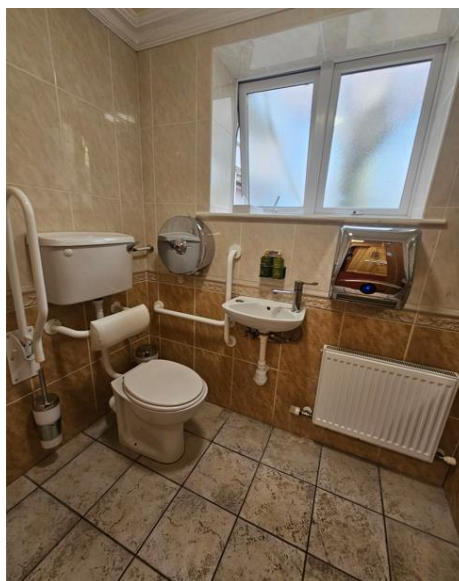
Public Area Accessible Toilet
