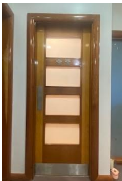
Ladies Changing and Toilet Entrance
